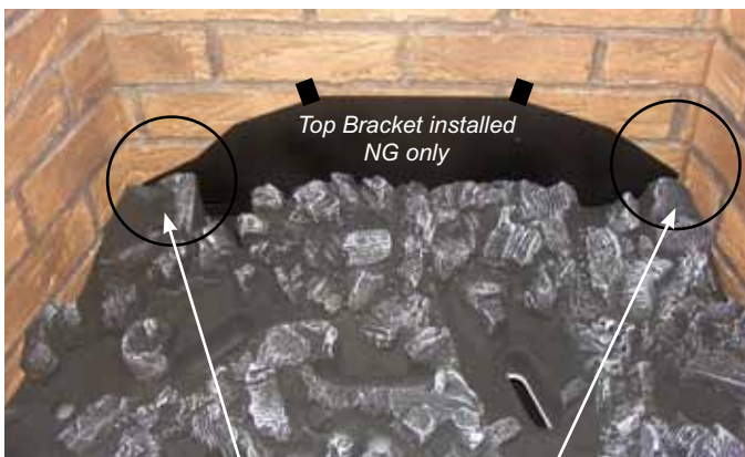
Log 1 provisions on burner tray
